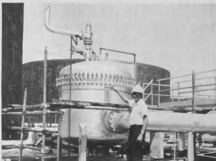
Camilo Daal of Mech.-Engineering shows one of 219 special filter cartridges contained in this milli-pore jet fuel filter unit. This new filter system helps assure maximum product cleanliness.
